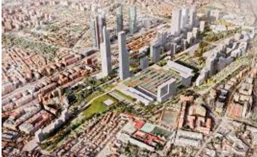
Figure 5 - Madrid's Charmartin HSR Station serves northern HSR lines and is being connected to Atocha Main Rail station via a new rail tunnel.
