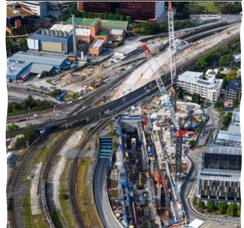
Brisbane-Gold Coast Line Upgrade under construction
