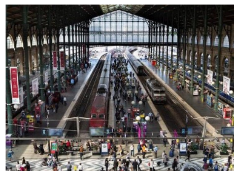
Gare du Nord station in Paris [1]
