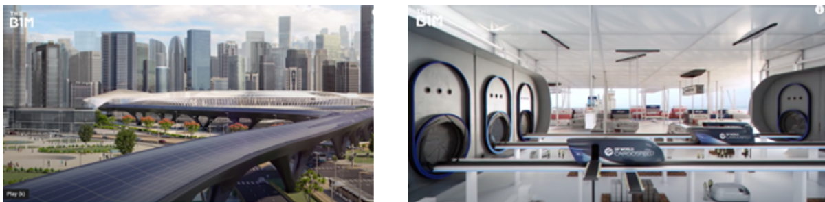
Hyperloop Station Concept. External view (left) showing raised guideway and station. Internal view (right) showing pods emerging from evacuated tubes [14]
